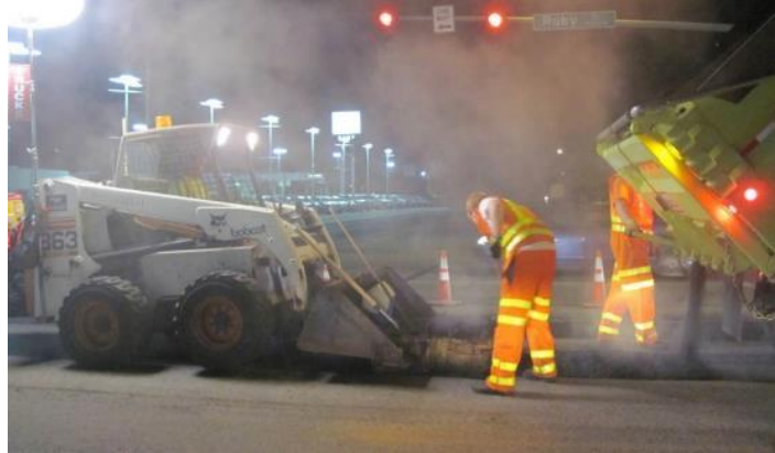
Maintenance patching pavement at an intersection requires significant planning, night work, and traffic control
