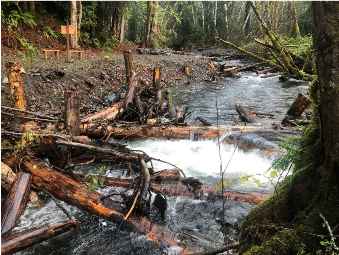
Figure 10-6 Example of Small-Channel Complex Log Grade Control
