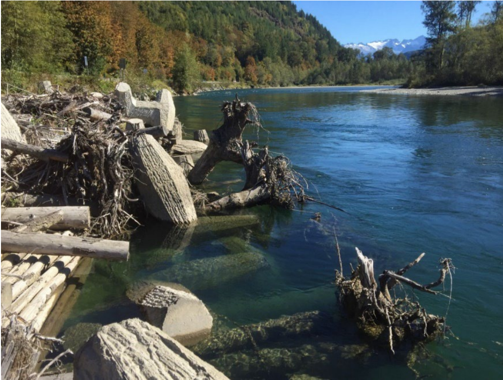
Figure 10A-9 Dolotimber Structures, Skagit River, Skagit County
