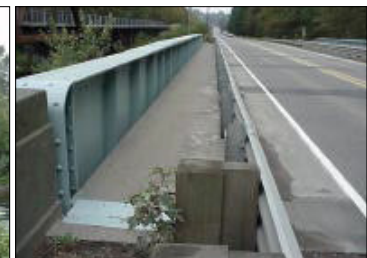
Elem #107 Steel Open Girder
