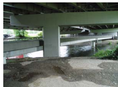
I-405 and pedestrian bridge crossing of the Cedar River
