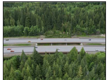
The MDT recommended building large bridges at many streams and known wildlife crossing areas. (Shown: Design visualization for two bridges at the wildlife corridor near Hudson Creek)
