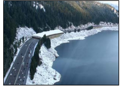
WSDOT modified the project design to eliminate the viaduct bridges and replace the existing snowshed with a new, larger structure. (Design Visualization)
