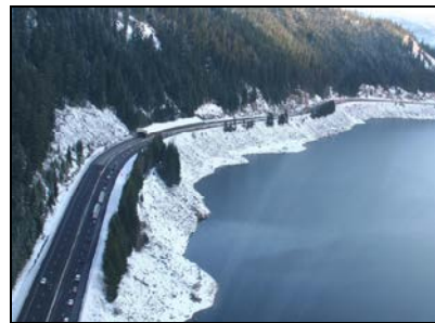
The existing snowshed does not adequately protect the roadway from avalanche danger.
