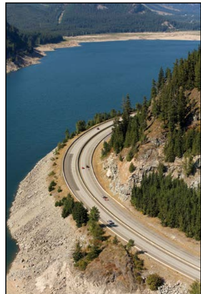
In some areas, terrain prevents WSDOT from treating stormwater.
