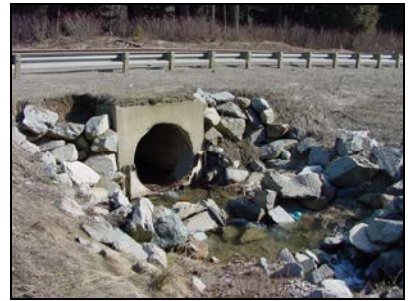
Many streams in the project area cross I-90 through narrow culverts. (Shown: Townsend Creek)
