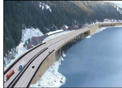
In the Draft EIS, Alternatives 2, 3, and 4 included viaduct bridges parallel to the shore of Keechelus Lake in front of the snowshed. (Design Visualization)
