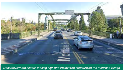
Decorative/more historic looking sign and trolley wire structure on the Montlake Bridge
