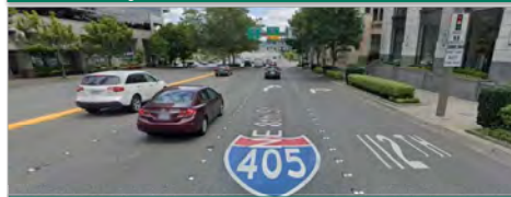
Painted directional shields on pavement on NE 8th St in Bellevue
