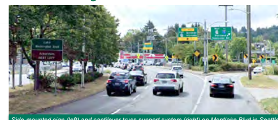
Side-mounted sign (left) and cantilever truss support system (right) on Montlake Blvd in Seattle
